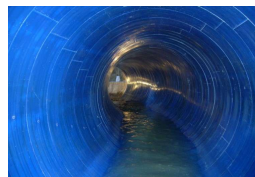
Pipeline rehabilitation (3S segment method)
