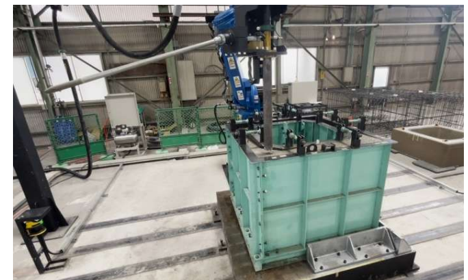
Concrete placement into 3D-printed formwork
