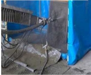
Mortar spraying method
