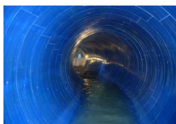
Pipeline rehabilitation (3S segment method)
