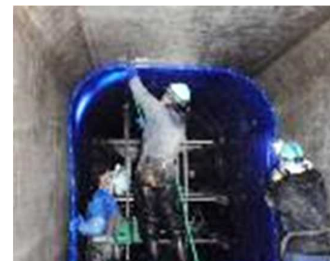
Rehabilitation work for Concrete Pipe
