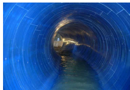
Pipeline rehabilitation (3S segment method)
