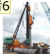
Pile installation
