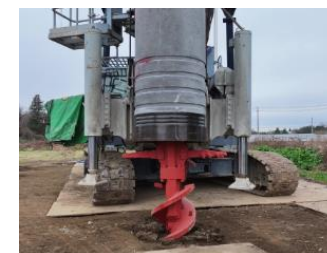
New inner excavation method (CP-X method)
