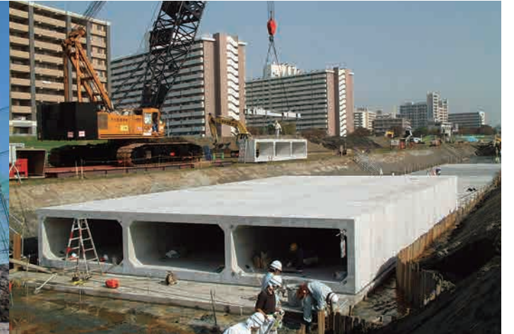
Box culvert (3,200×1,250mm; Triple-line)
