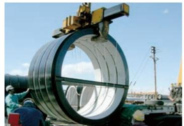
外圧強さ:1種~6種／内圧強さ:0.6MPa~1.2MPa
